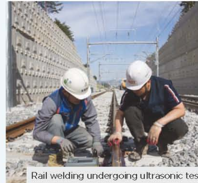
Rail welding undergoing ultrasonic test
