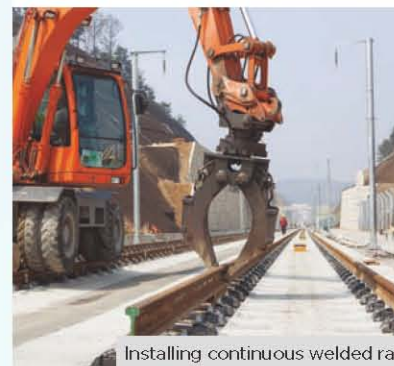
Installing continuous welded rail
