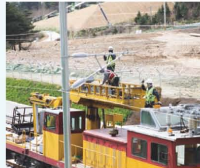
Clamping of contact and messenger wires
